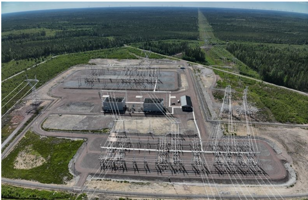
Picture Pyhäjoki Valkeus 400/100 kV substation
